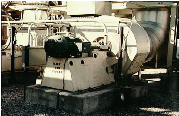
Figure 1. Fan (background) and drive motor (foreground, EPRI)
